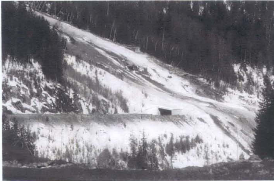
Figure 5. A snow shed protecting the Trans-Canada Highway at Rogers Pass, British Columbia. Photographer: C. Stethem.
