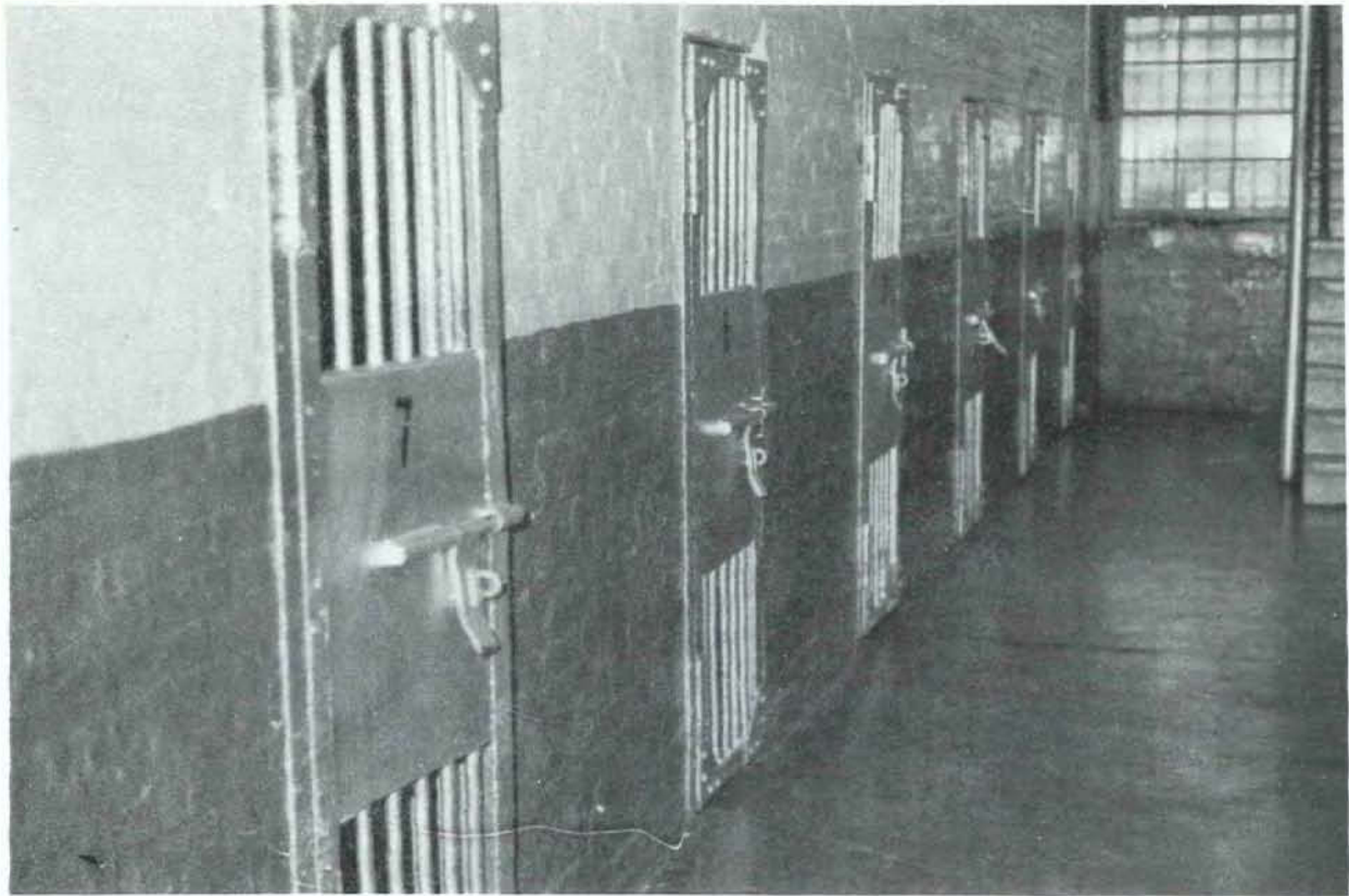
Main Cell Block: Queens County Jail
