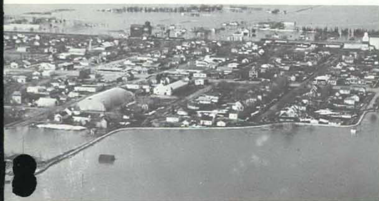
Perimeter diking (foreground) at Morris
