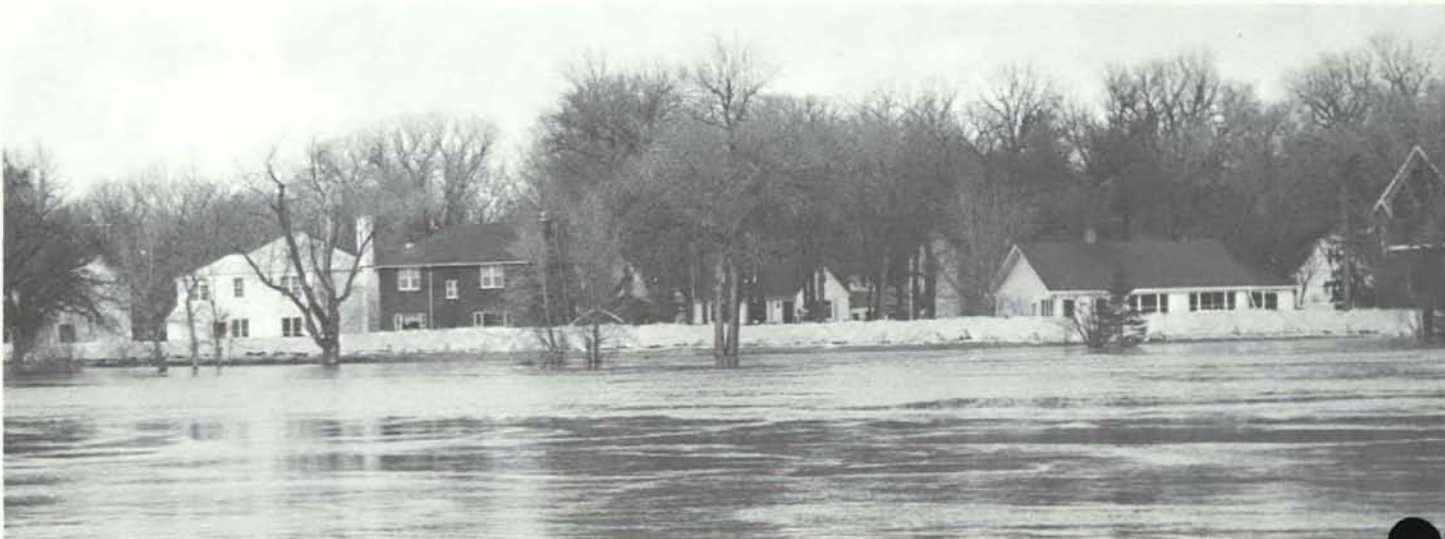
Secondary diking with Red River in foreground
