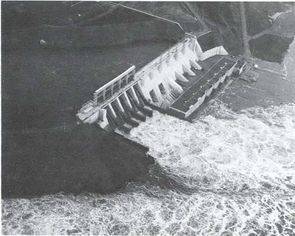
Mactaquac Dam is allowing the St. John River to run naturally—the 10 gates are open. The River experienced the greatest flow since records began to be kept in 1918. The flow is at least 50,000 cu. ft. per second—higher than anything in the records.
