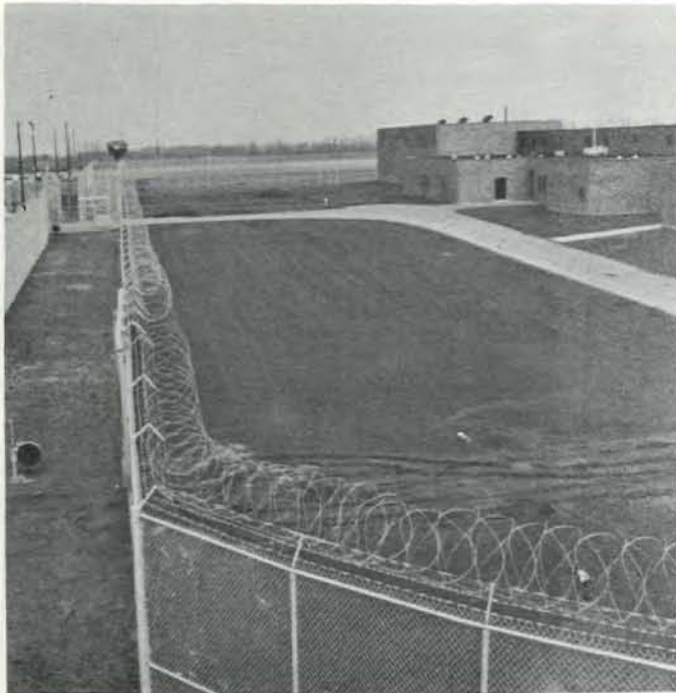
Edmonton Institution, opened in 1978, utilizes both an electronic surveillance system, and staff and towers to maintain its security.
