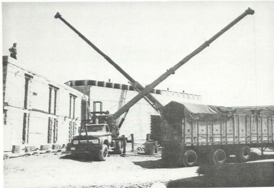
The exterior of the new accommodation building
