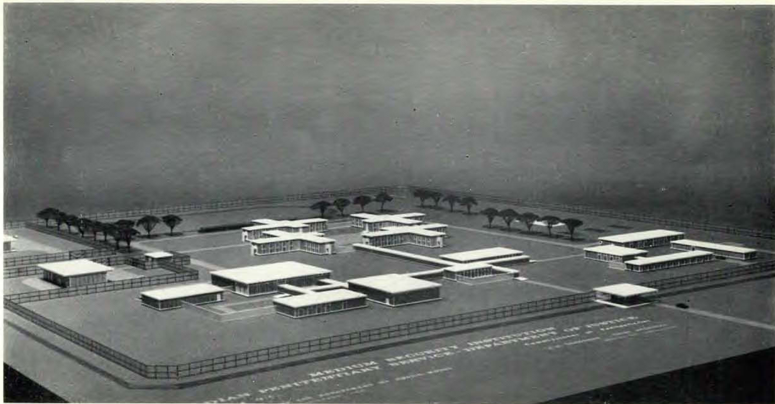
The Standard Medium Security Institution of the Canadian Penitentiary Service. This photograph illustrates the buildings comprising a Medium Security Institution of which a number are either under construction or to be constructed at various locations in Canada. Each institution will accommodate 467 inmates. The planning of the institution was based on the concept of 5 "centres", i.e., groups of buildings to which an inmate goes for appropriate purposes at different times during the normal day.
